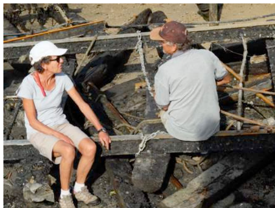
Pam and Bruce at Davis Marina – slipway rebuild and clean up
